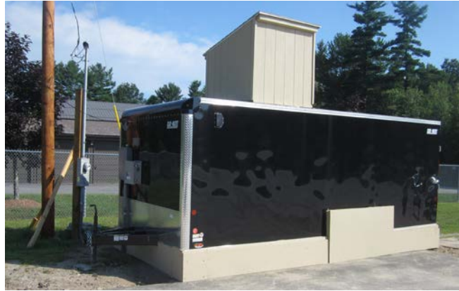
Figure 5. Transportable bioreactor in Auburn. Insulated to protect the biomass from New Hampshire winters.
