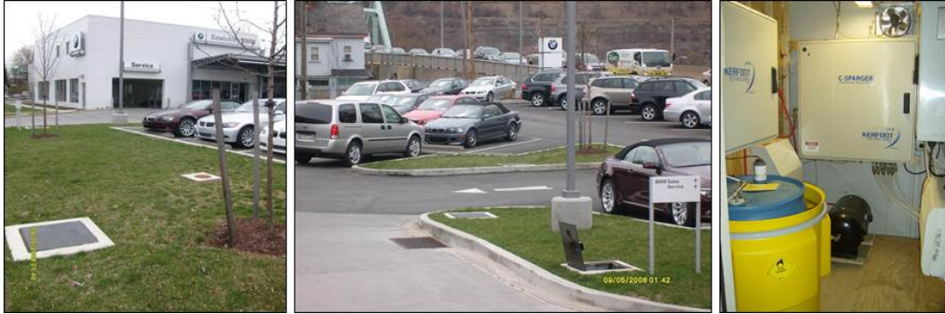
Figure 8. Minimally Invasive Installed Perozone™ System - As-Built Photographs.
