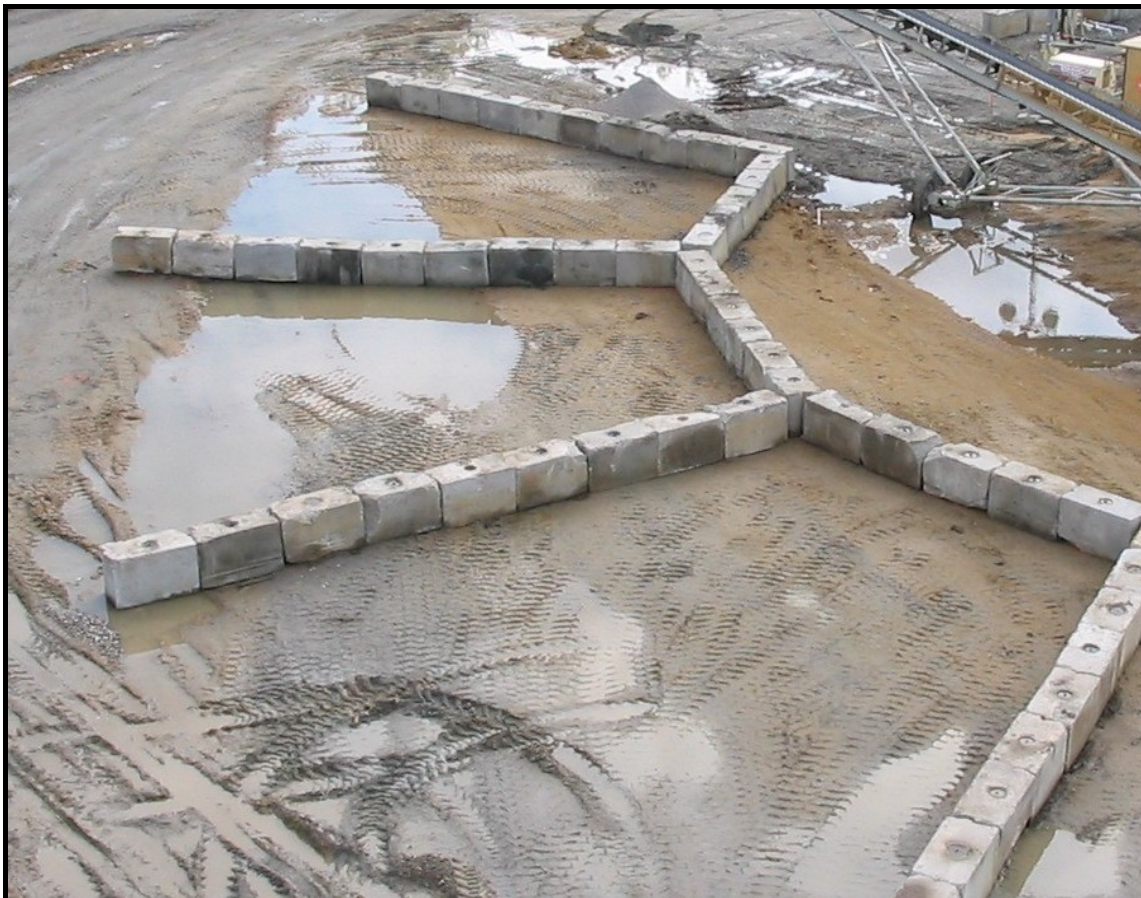
Figure 6. Site Infra-structure designed for 500 cy piles
