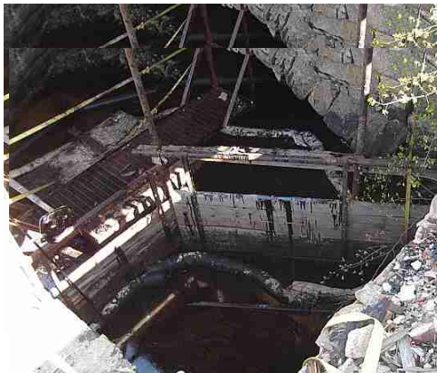
Figures 35 and 36. Channel diversion wall installed in 2005 to direct canal water away from the oil-impacted western tailrace.
