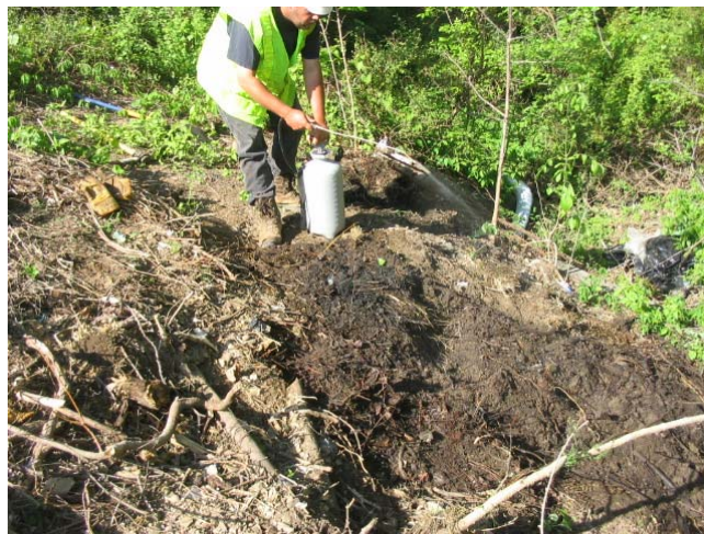
Figure 2. Application of AgroRemed to impacted soils
