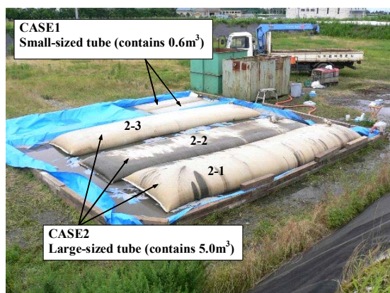
Photo 1. View After Execution
