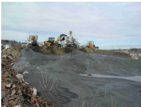
Figure 31 (left). Application of flowable fill to encapsulate debris. Figure 32 (right). Flowable fill after setting and curing.
