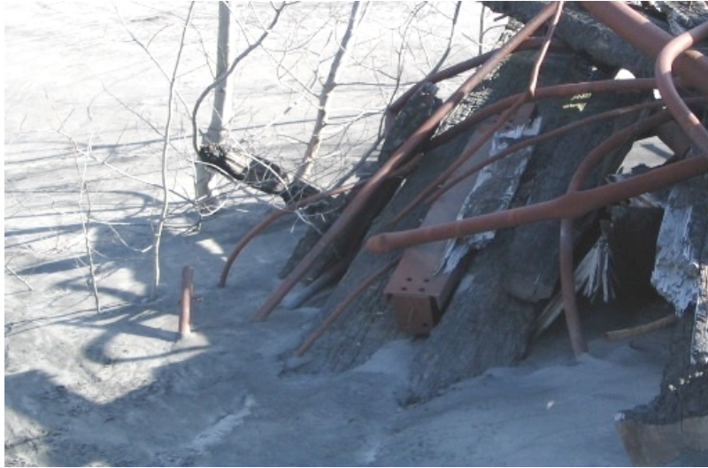
Figure 30. Encapsulation of debris with flowable fill.
