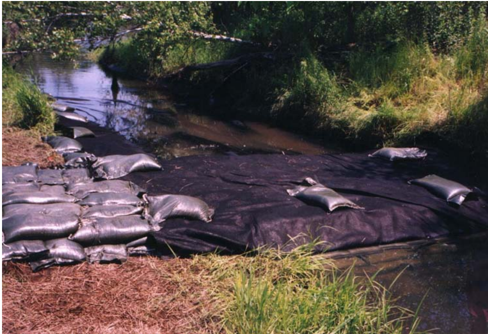
Figure 15. Sand bag dam installed in June 2002.
