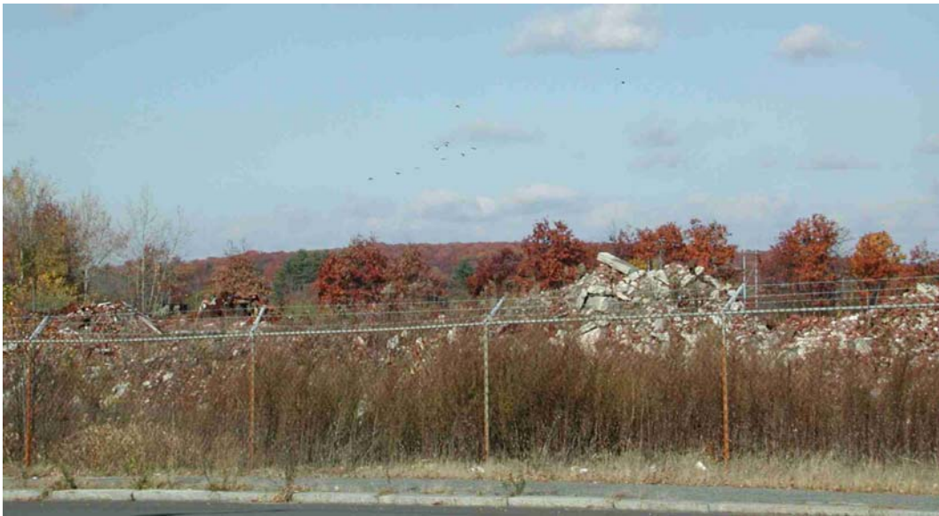
Figure 28. Fisherville Mill Site before encapsulation with flowable fill.
