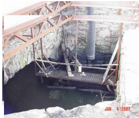
Figures 35 and 36. Channel diversion wall installed in 2005 to direct canal water away from the oil-impacted western tailrace.
