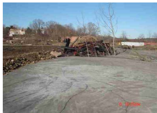
Figure 31 (left). Application of flowable fill to encapsulate debris. Figure 32 (right). Flowable fill after setting and curing.
