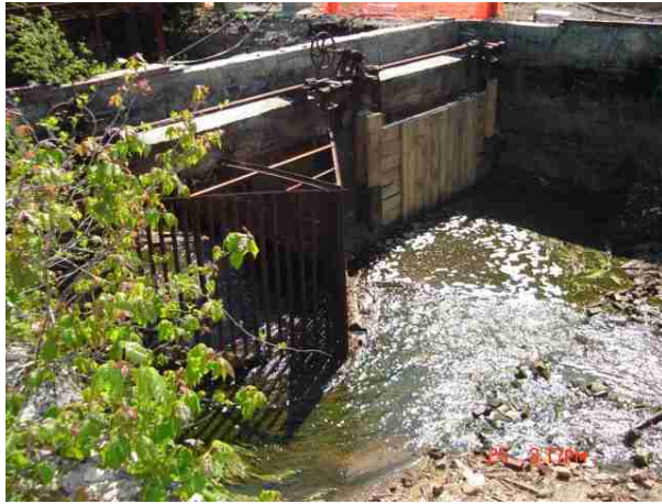
Figures 35 and 36. Channel diversion wall installed in 2005 to direct canal water away from the oil-impacted western tailrace.
