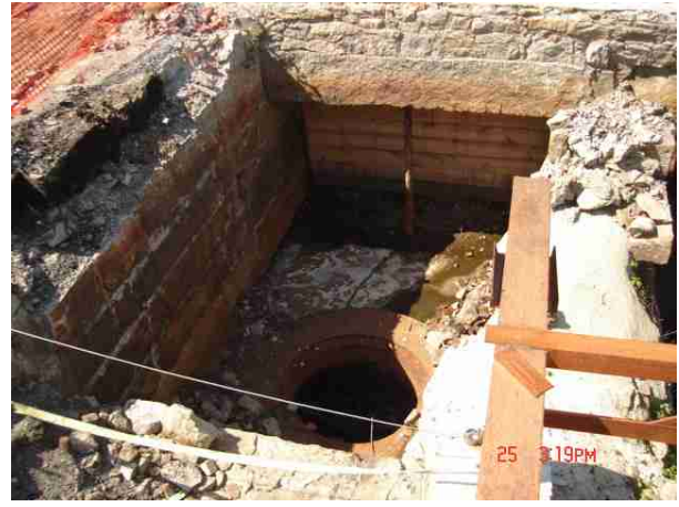
Figures 35 and 36. Channel diversion wall installed in 2005 to direct canal water away from the oil-impacted western tailrace.
