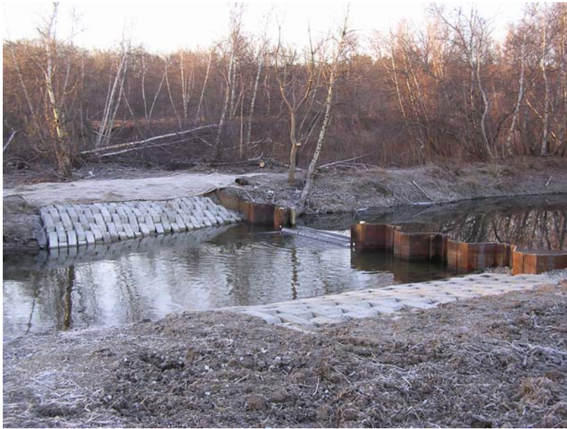
Figure 16. Sheet-piling dam installed in December 2003.
