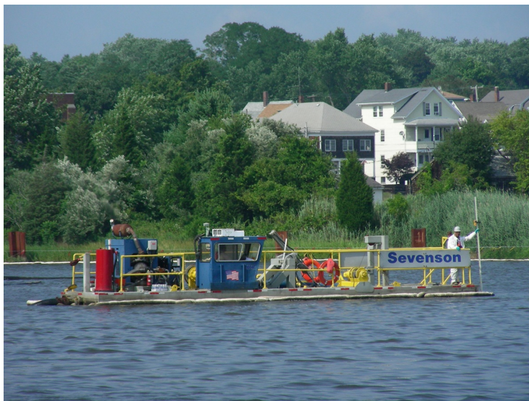
Figure 3. Dredging New Bedford Harbor.
